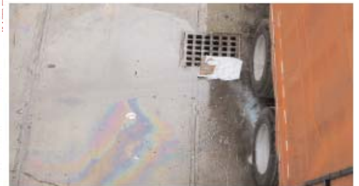
This oil sheen, left by parked vehicles, makes its way towards this catch basin and storm drain network. Without proper treatment, the oil will enter the nearest surface water, where it will degrade fisheries habitats.
